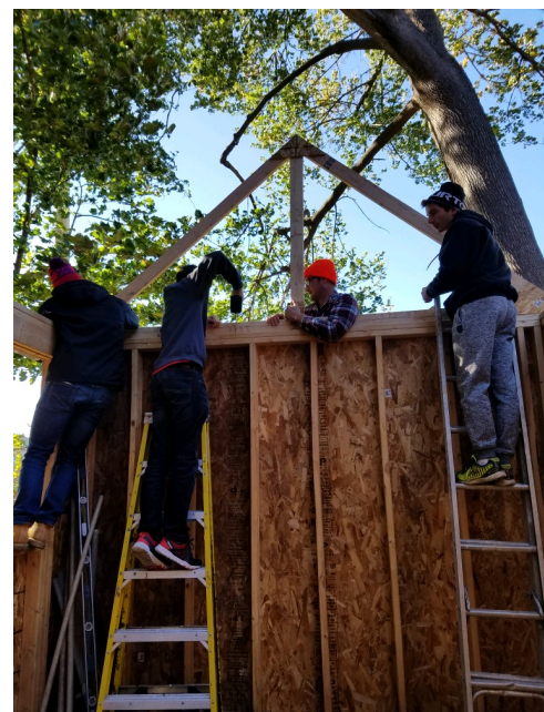
The new shed, a work in progress
